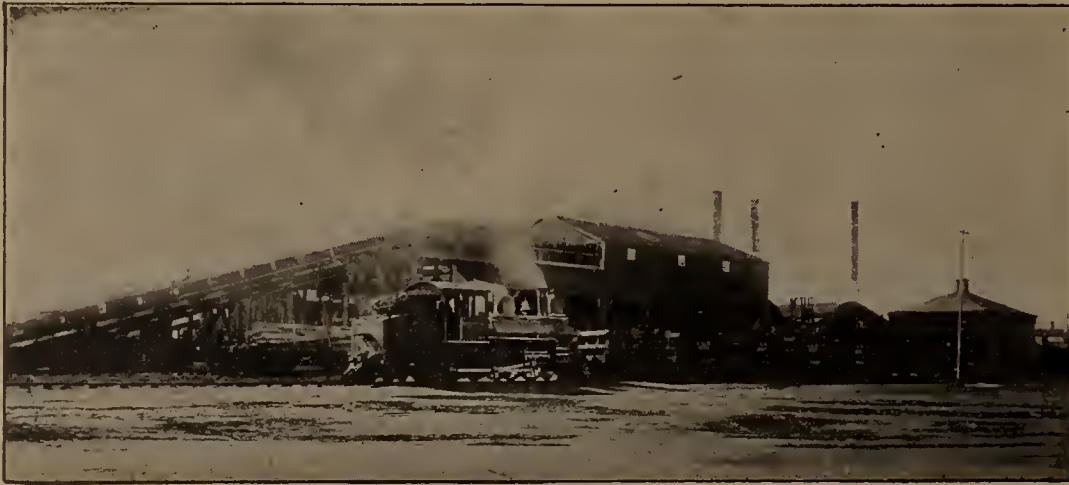
COLLIERIES AT WESTVILLE, NOVA SCOTIA.
